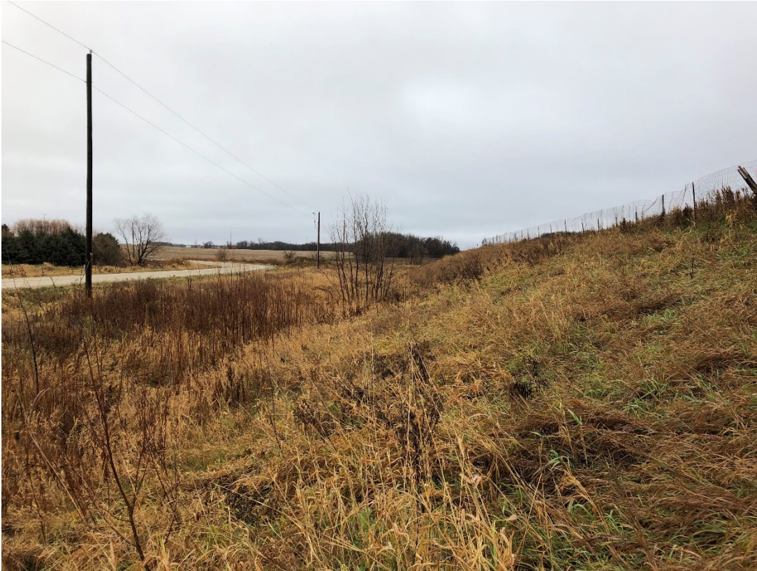
Photo 27: Location 9 – Looking South, Phase 2 Eastern Berm
