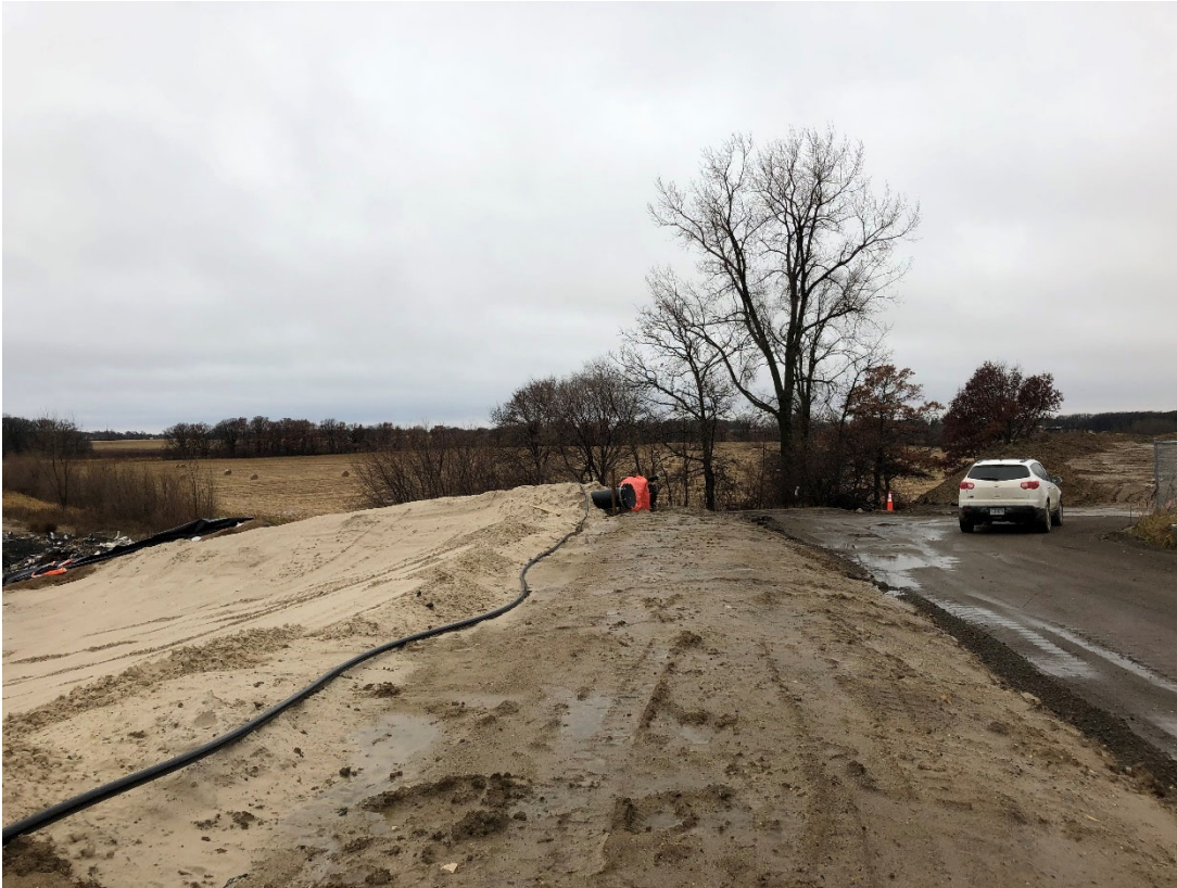
Photo 3: Location 1 – Looking Southwest, Phase 4 Anchor Trench
