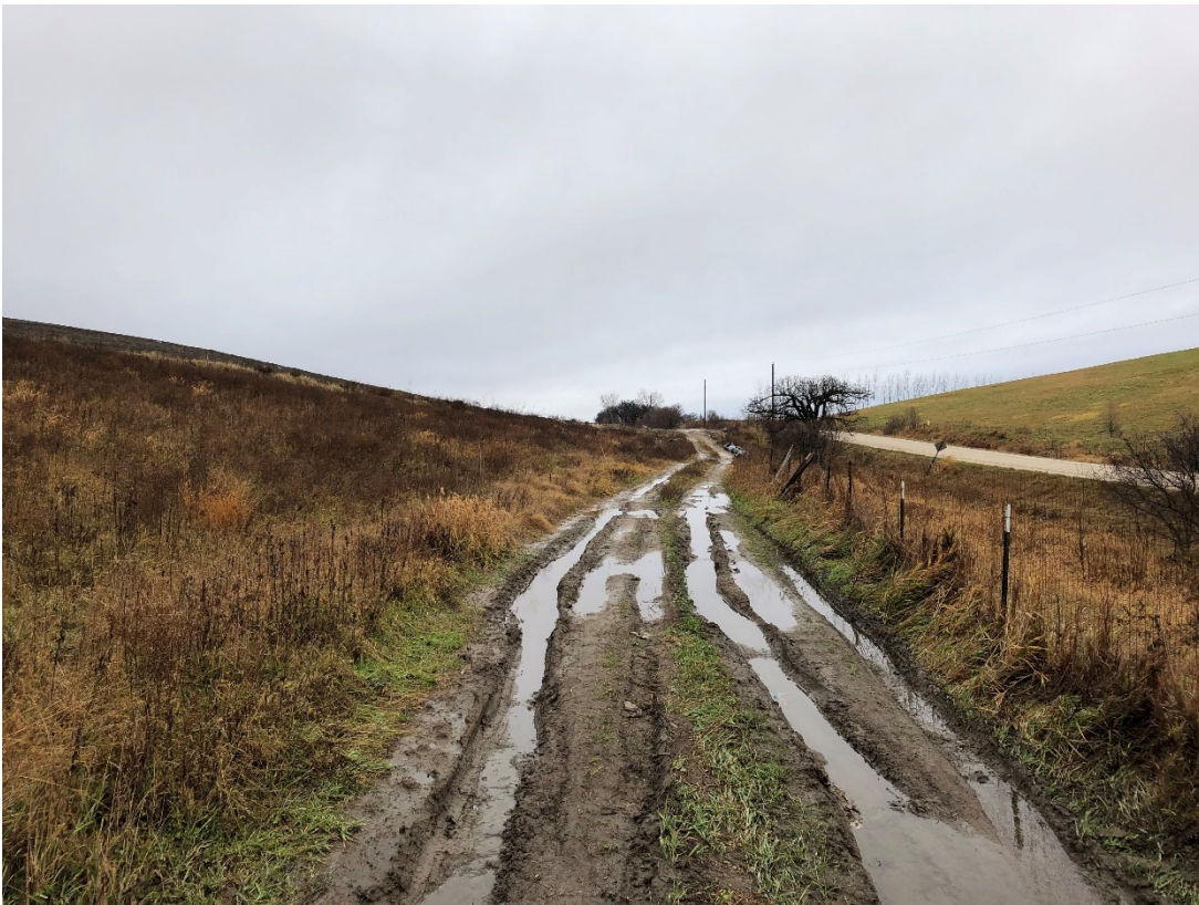
Photo 26: Location 9 – Looking North, Phase 2 Eastern Perimeter Road & Slope
