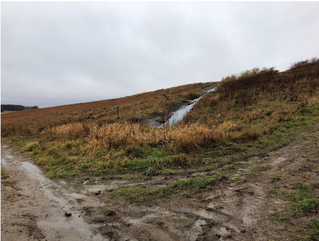
Photo 14: Location 6 – Looking West, Phase 1/2 Overlay Liner & Southern Slope
