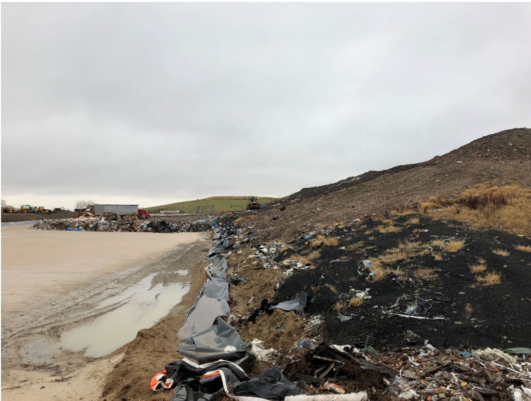
Photo 6: Location 2 – Looking East, Phase 4/3 Connection & Phase 3 Northern Interior Slope
