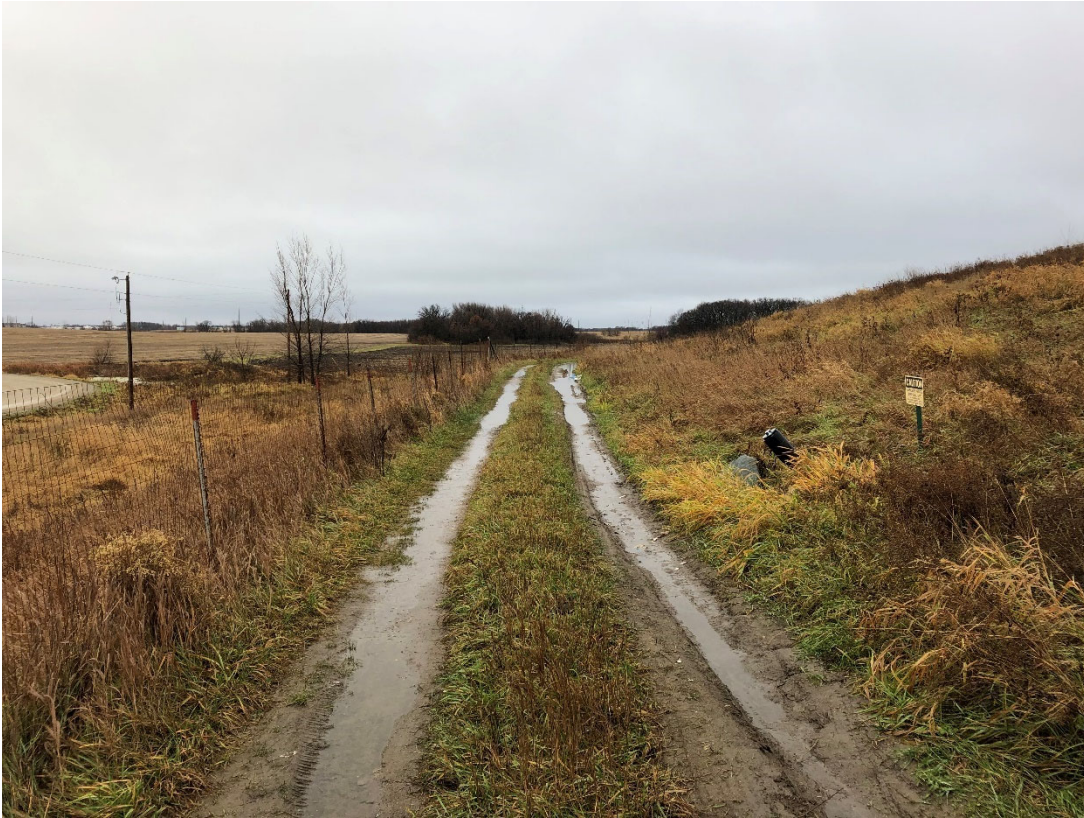
Photo 25: Location 9 – Looking South, Phase 2 Eastern Perimeter Road & Slope
