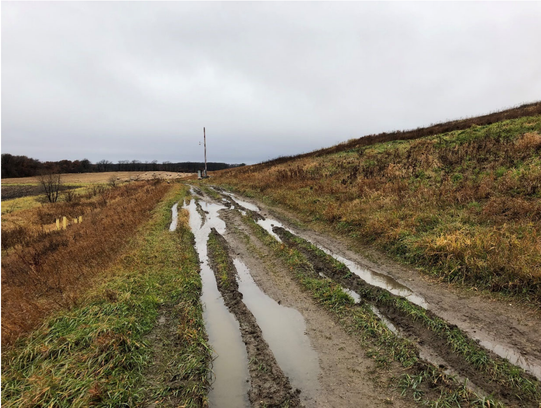
Photo 17: Location 7 – Looking West, Phase 2 Southern Perimeter Road and Slope
