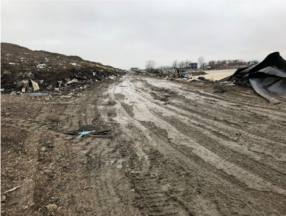
Photo 31: Location 11 – Looking West, Phase 3/4 Connection, Phase 3 Norther Interior Waste Slope
