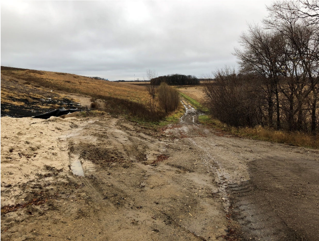
Photo 5: Location 2 – Looking South, Phase 3/1 Western Perimeter
