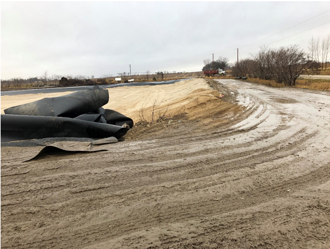
Photo 32: Location 11 – Looking North, Phase 4 Eastern Anchor Trench
