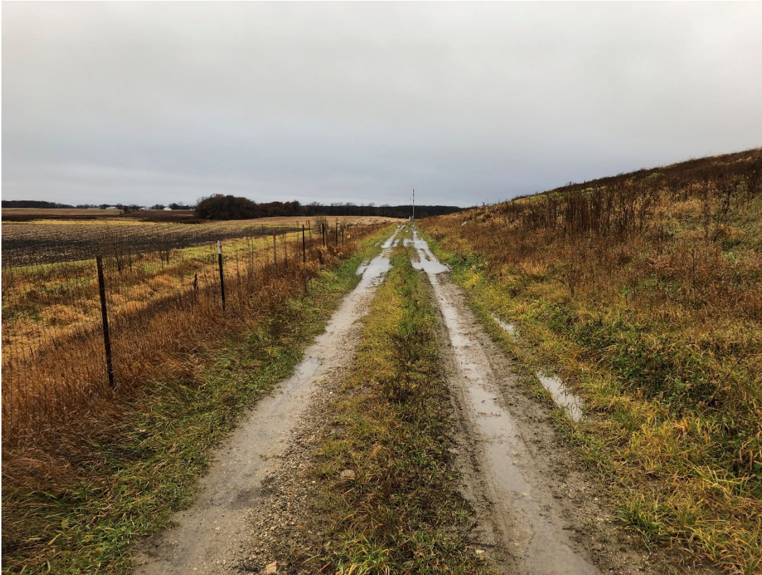
Photo 21: Location 8 – Looking West, Phase 2 Southern Perimeter Road and Slope
