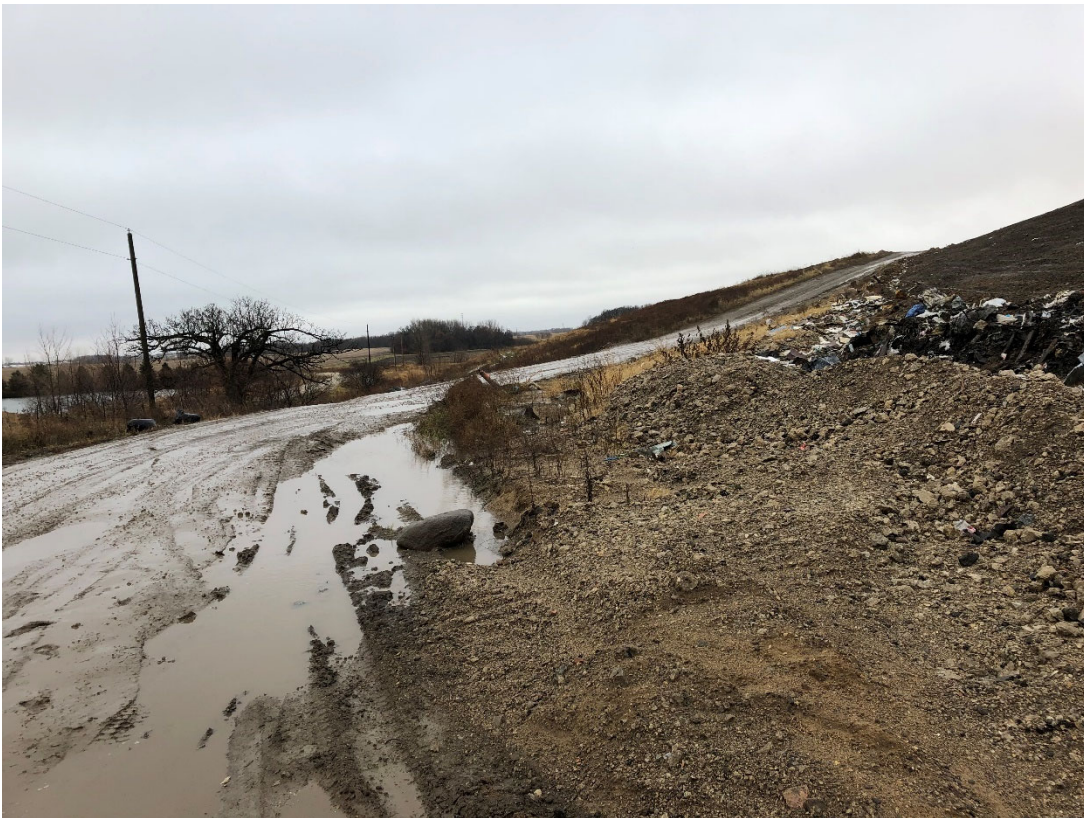
Photo 30: Location 10 – Looking South, Phase 2 Eastern Slope and Interior Access Road Entrance
