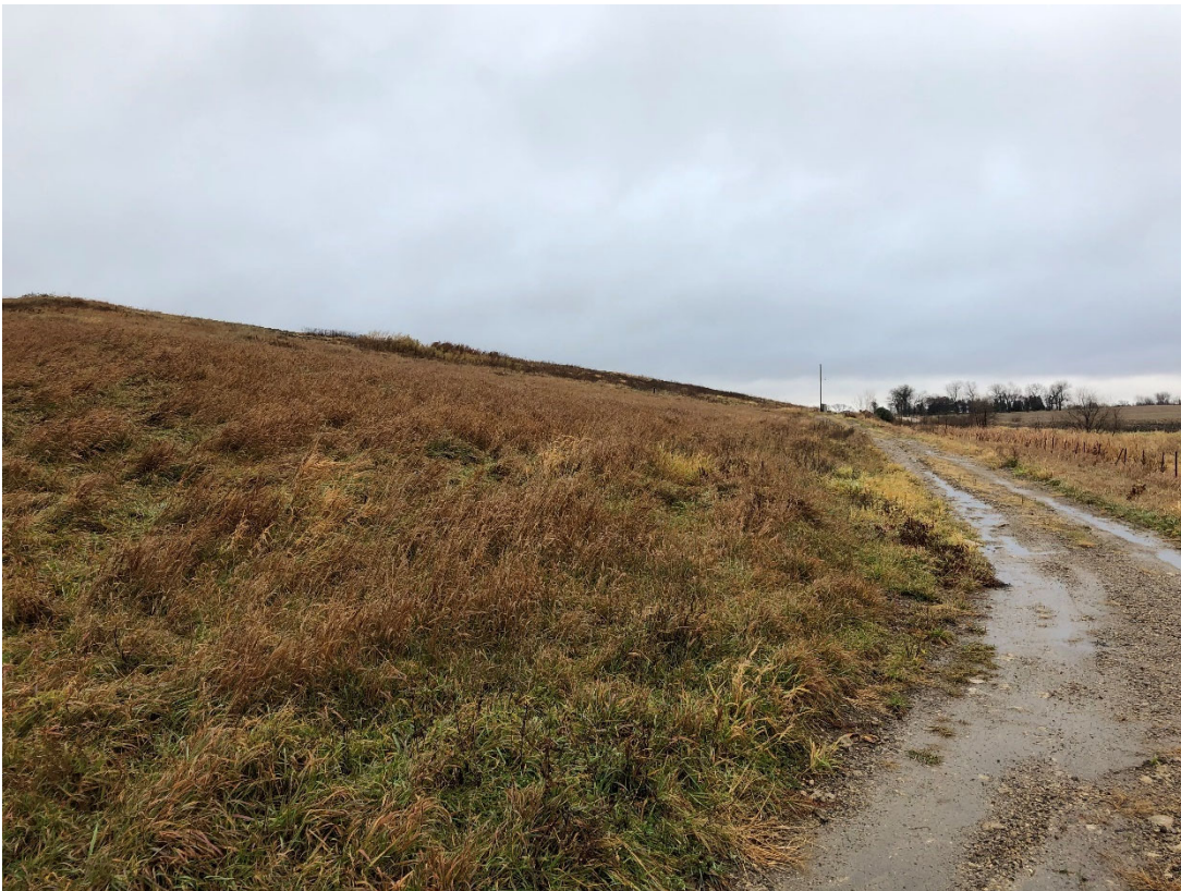
Photo 10: Location 4 – Looking East, Toe of Phase 1 Southern Slope
