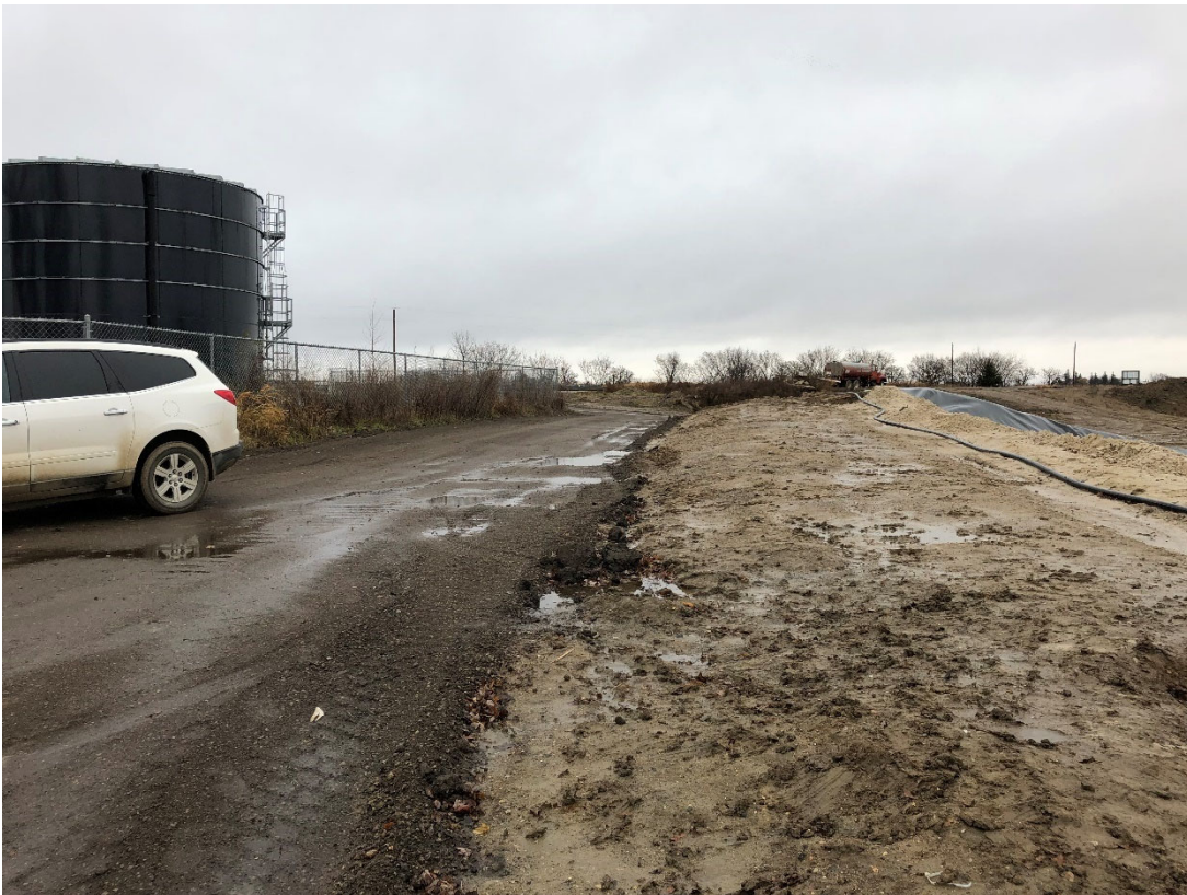
Photo 4: Location 2 – Looking Northeast, Phase 4 Anchor Trench
