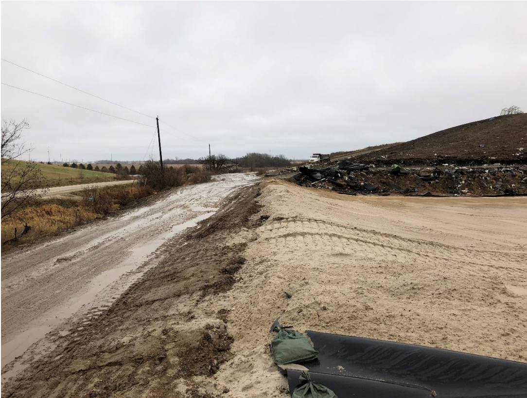
Photo 33: Location 12 – Looking South, Phase 4 Eastern Anchor Trench & Phase 3 Eastern Waste Slope
