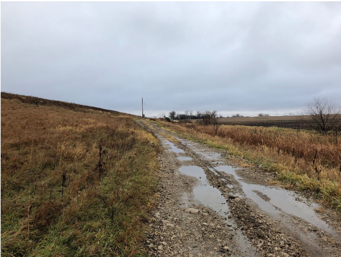
Photo 12: Location 5 – Looking East, Toe of Phase 1 Southern Slope
